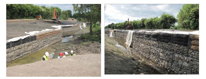
**Solution:** The original idea was to use the soxx as part of the remediation model however because the silt was highly contaminated with Nickel, Zinc, Copper, Arsenic etc. A Filter system was required to prevent contamination. The use of Filtrexx as a filter, given the solidification technique and the membrane was therefore no longer a primary focus of their use and the role of Filtrexx became more significant in terms of establishing vegetation and softening the look of the gabion wall.
